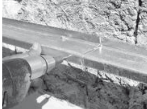
Connection of Z50 profiles, overlap 100 mm
