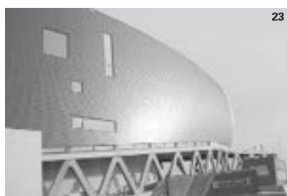
Photo 6 Administrative building SPORTEN, Nové Město, Czech Republic CETRIS® BASIC, façade cladding, VARIO system
