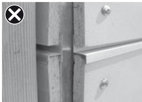
Diagram of zinc-coated profile installation for boards widths > 1,875 mm
